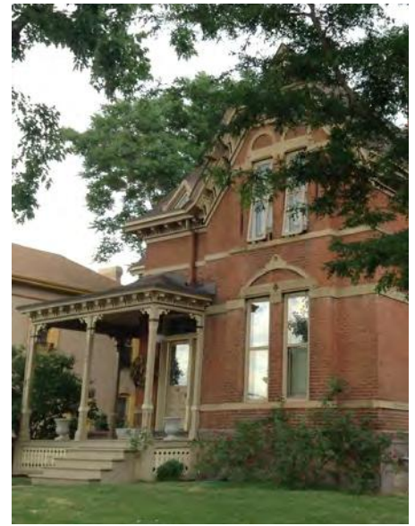
6. Elaborate Italianate style single family residence on Glenarm St. Note the stone foundation and brick walls, the projecting offset front porch and entry, the tall, narrow wood windows with elaborate headers and sills, and the heavy decorative cornice.
