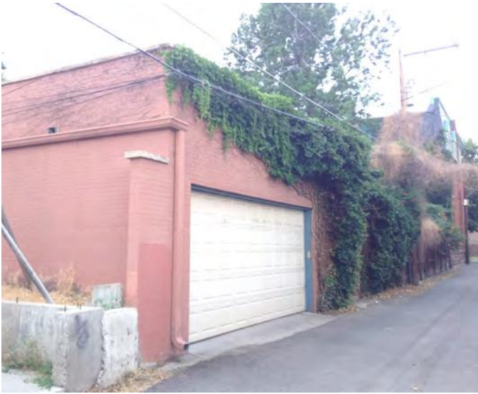
7. Carriage house structures within Clements Historic District. Accessed from the alleyway, one-story in height and of brick construction with a flat roof.
