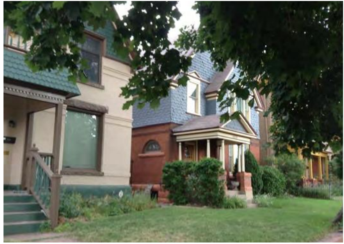
2. Glenarm Pl. streetscape. Note the uniformity in the front yard setback, the brick buildings with fish scale shingle in the upper stories, and projecting front porches of these Queen Anne style structures.
