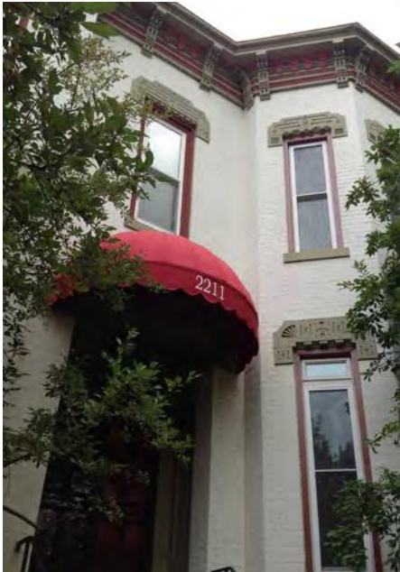
4. Italianate style rowhouse on Glenarm Pl. Note the heavy roof cornice, elaborate window headers, and tall narrow windows.
